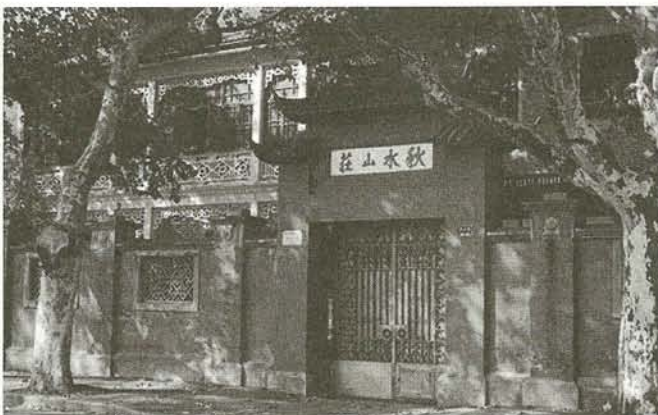
Autumn Water Mountain Pavilion, before restoration.
